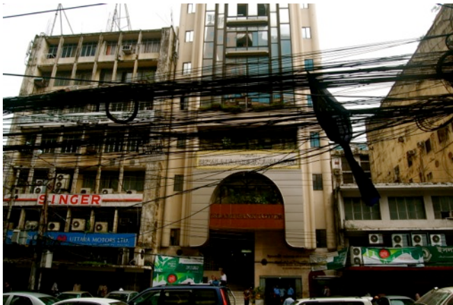
The Islami Bank Bangladesh Limited headquarters, Dilkusha, Dhaka, Bangladesh (2010)
