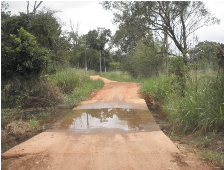
Figure 2: Poor road conditions
